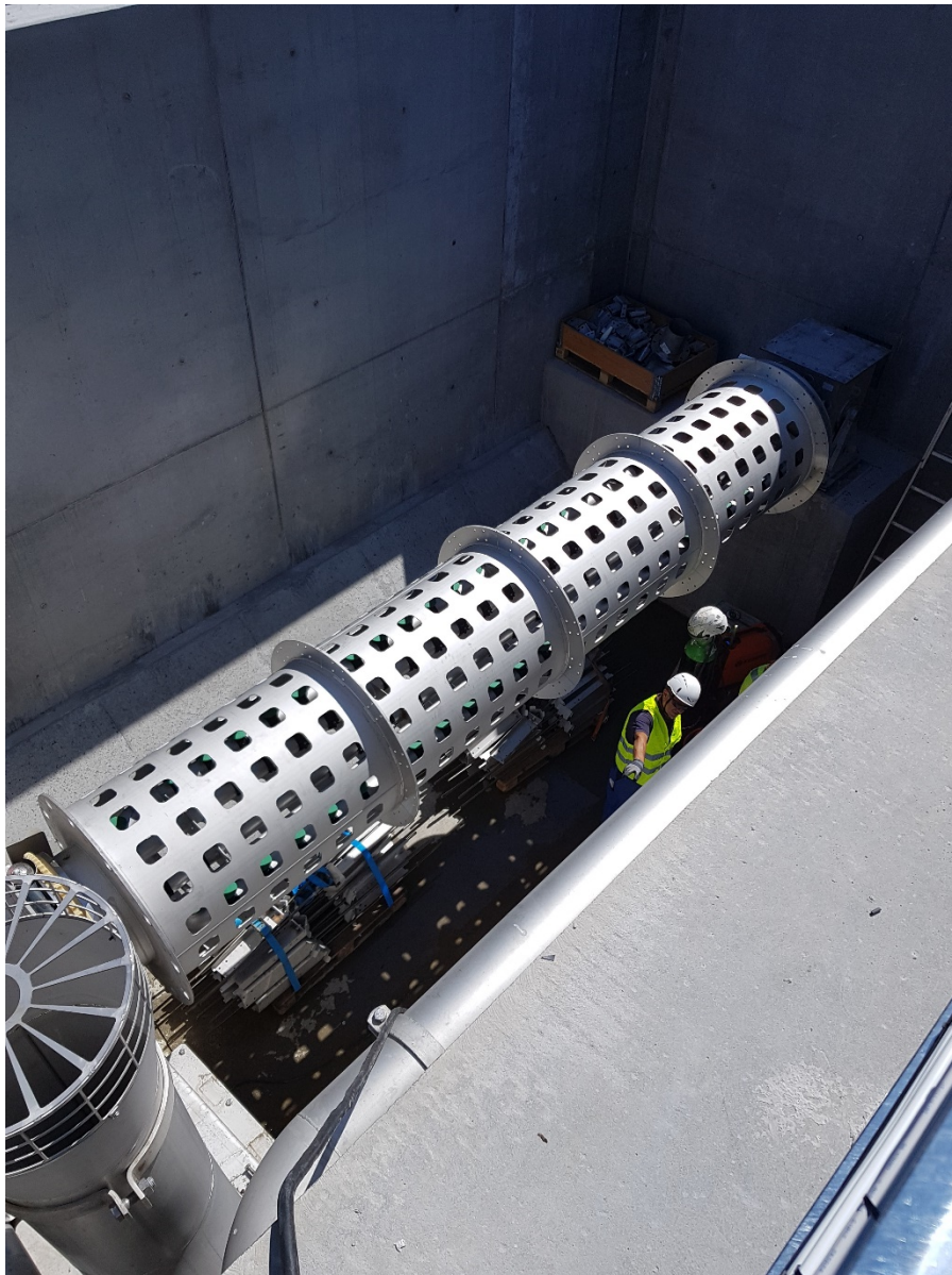
Montage membranfilter.
